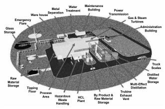
Fig. 3: The Multi Activity Waste to Energy Complex (Source: Energy Planet)
