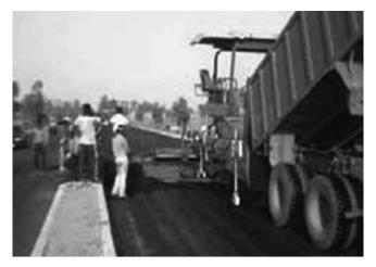
Fig. 4: Laying of Plastic Waste Modified Mix at Rohtak-Bhiwani road
