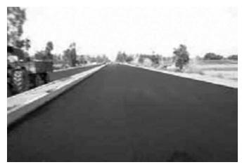
Fig. 5: Finished Surface of Plastic Waste Modified Mix at Rohtak-Bhiwani Road
